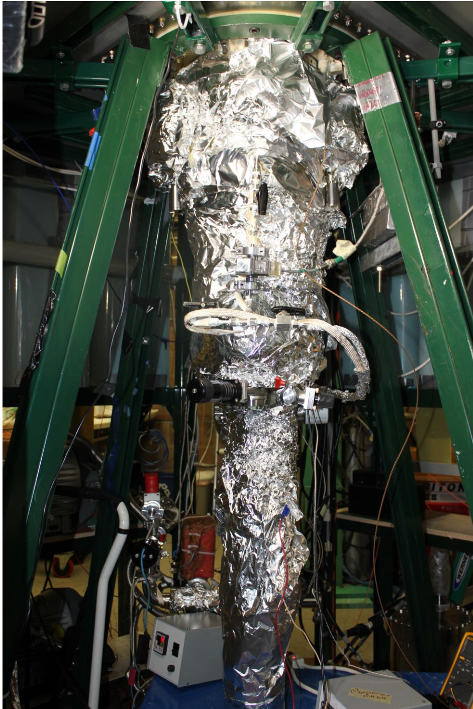
Figure 11. The FF-2B vacuum chamber with insulation and outer aluminum foil. Now it looks like a baked potato, but getting the bake-out done is more important than looks!
